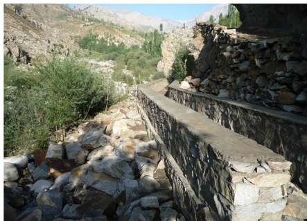
Construction d'un canal, Naw Safa CDC, Kunar
